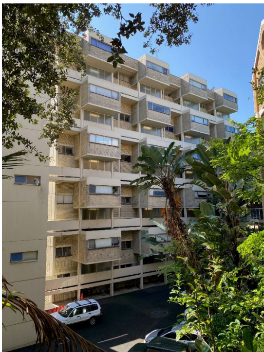
Figure 1 Aquarius (1965), Rushcutters Bay, was the first and most comprehensive project where Seidler explored split-level planning, as found in the northern building of Ercildoune. (Source: GML)
